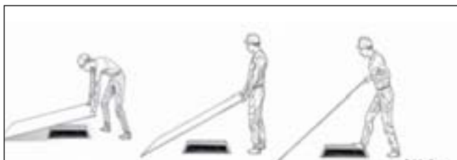
Figure 1. This roofer does what many have done. Pick up the plywood. Walk it forward. And step into a hole. (Courtesy of Ellis Fall Safety Solutions, www.FallSafety.com )
