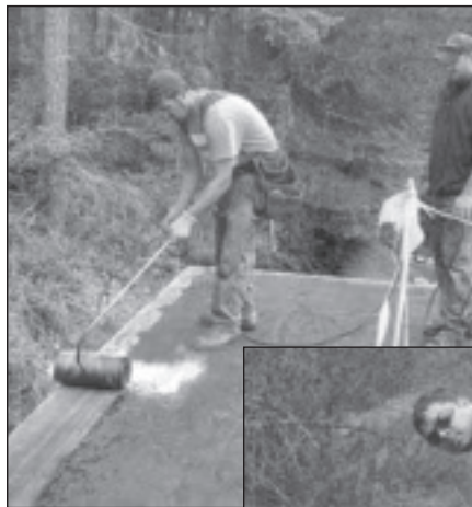
Apprentice Blake Stokke applies torch-down material while supervised by Ryan Weichert.
