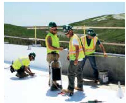
Installing cap sheet at Marine Drive, with Mount Hood in background.
