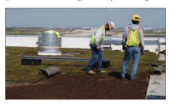
Roofer's Local 11 members roll out plant mats on a new vegetative roof in the Chicago area. A vegetative roof is still a roof. So it is best installed by skilled union roofers.
