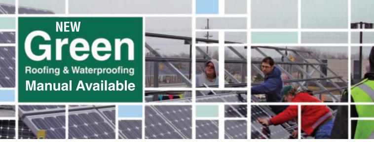
Roofers Local 26 members work with electricians to install PV panels on a municipal building in Indiana. Roofers ensure the integrity of the roofing system and leave the BOS (Balance of System) electrical connections to the electricians.
