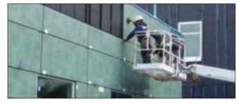
Exterior panels are placed over a green air/vapor barrier by Roofers Local 81 members on this new building at Marin College in the San Francisco Bay area. Roofers and waterproofers installed the air/vapor barrier and the panels, which are important parts of the green building envelope.
