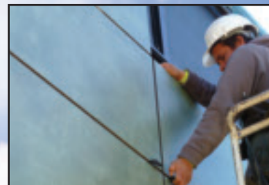
Foreman Jose Martinez carefully attaches the Trespa panels to the vertical bars with the spacers set to specification.
