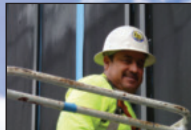
Jesus Garcia takes a well-deserved break and poses for the camera after installing vertical bars.
