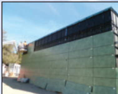
Miguel Perez and Jesus Garcia attach Trespa panels from a boom lift at College of Marin.
