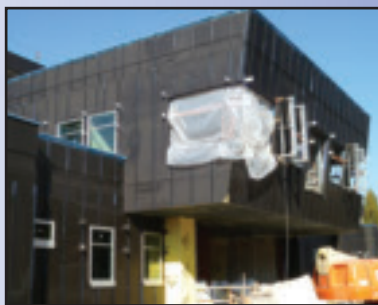
The front entrance to the Science Building project at the College of Marin. The exterior of the building was sprayed by our roofers with Henry Air-Bloc 33 as an air barrier. Vertical bars were then attached to the building to hang the Trespa panels on.
