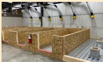
EPDM and hot-air welding mock-ups have extra ventilation.
