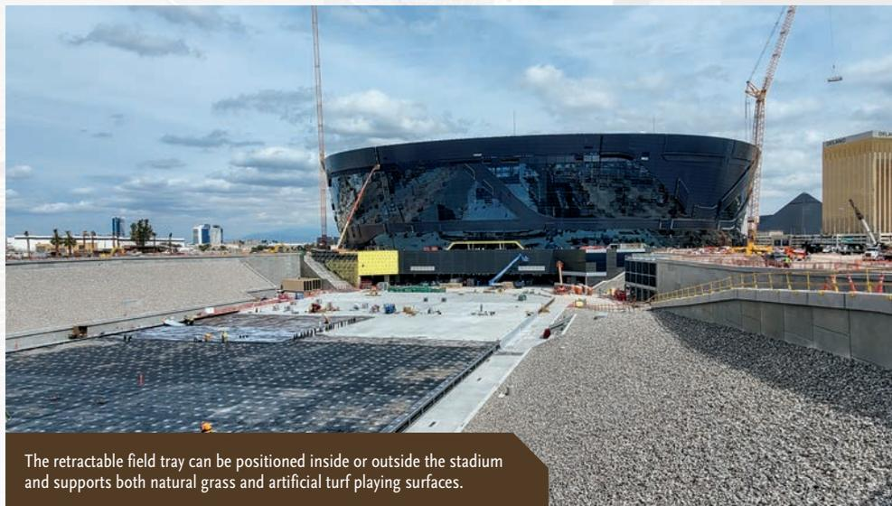
The retractable field tray can be positioned inside or outside the stadium and supports both natural grass and artificial turf playing surfaces.
