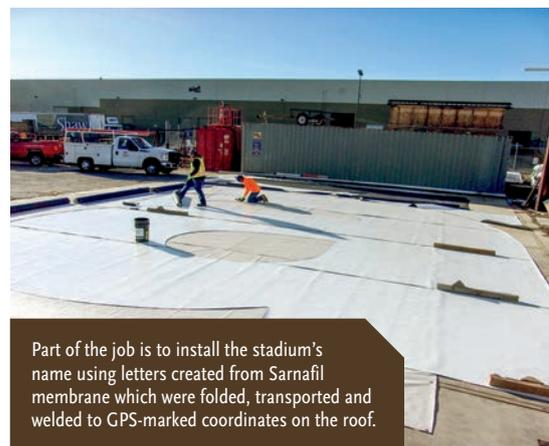
Part of the job is to install the stadium's name using letters created from Sarnafil membrane which were folded, transported and welded to GPS-marked coordinates on the roof.
